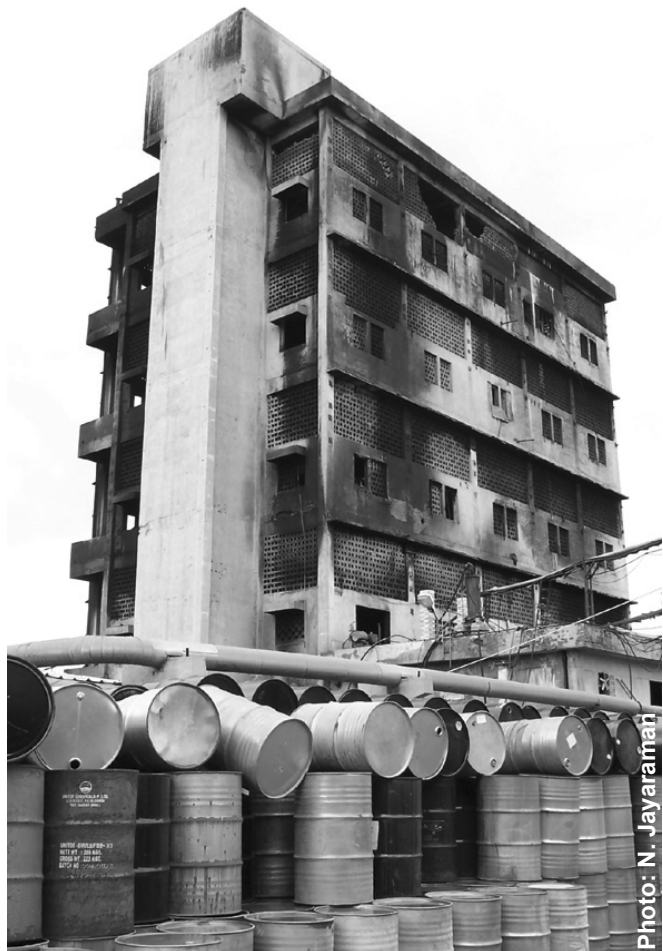
The Burnt Endosulfan Plant
